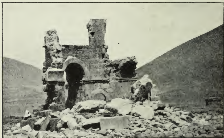
FIG. 59.—Interior of No. 8, from S.-W.
